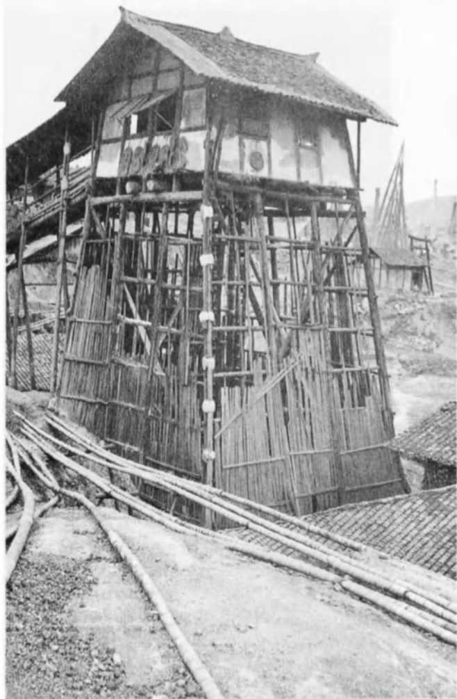
Well-head and derricks photographed over 40 years ago in Sichuan Province. In foreground, the traditional bamboo pipes which led the natural gas to nearby towns.
